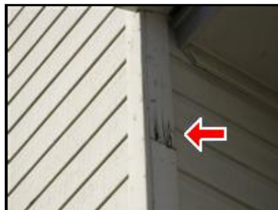
E. Picture 17 Chimney trim below upper roofline
