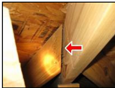
D. Picture 7 Right rear of home
