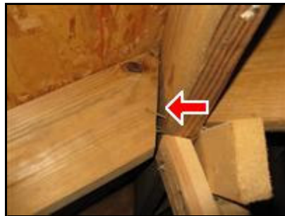
D. Picture 5 Left front of home
