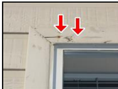
E. Picture 15 Rear window beside fireplace
