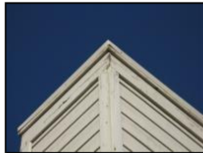
E. Picture 8 Weathered chimney trim
