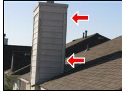
E. Picture 12 Weathered trim needs sealing
