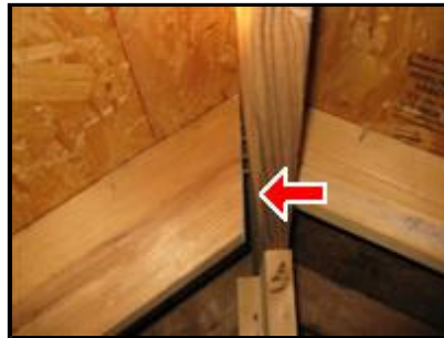
D. Picture 3 Left front of home
