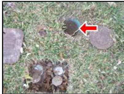
Shutoff valve buried
